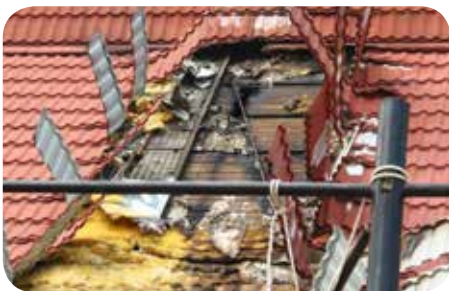
TMC roof damaged by fire (2003).
