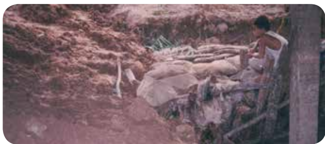
Sandbags shoring up the beams of Takhmao Trinity Methodist Church (2002).
